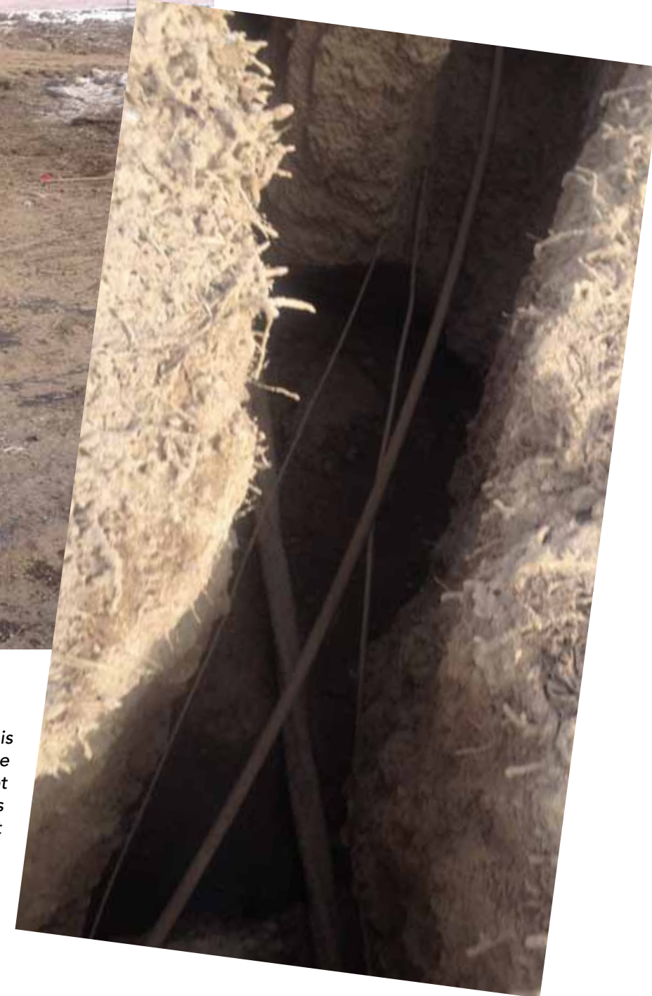
Exposing entire spans of buried cables in a right-of-way.
